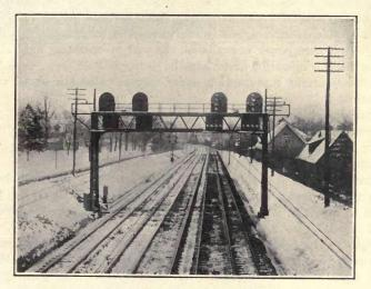
FIG. 6 .--- Position-light signal.
