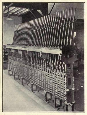
FIG. 36.-Style A interlocking machine.
