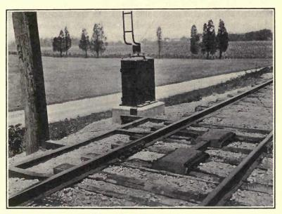
FIG. 245.-Impedance bonds in place.
