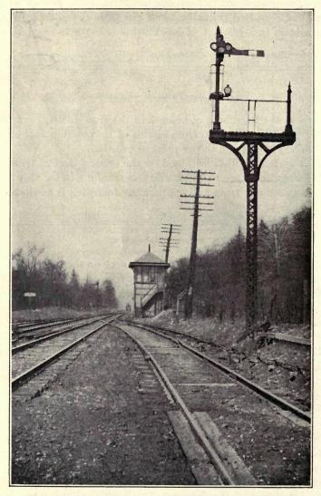
FIG. 218.—Absolute signal. (Hall Switch and Signal Co.)
