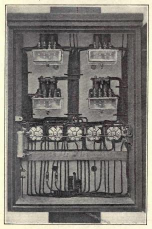
FIG. 173.—Lightning arresters in relay box.
