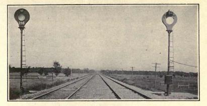
FIG. 7.-Disc signals arranged for left-hand running.
