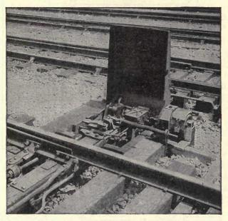
FIG. 121.-Model 2 switch machine.
