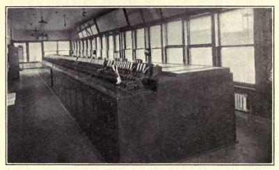
FIG. 145.—Federal interlocking machine.
