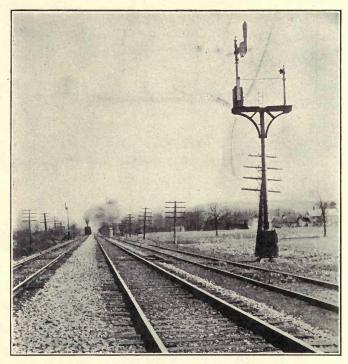
FIG. 14.-Bracket signal and doll post.
