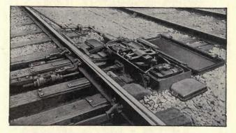
FIG. 124.-Model 4 switch machine.
