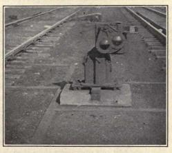
FIG. 15.-Upper quadrant two-position dwarf signal.
