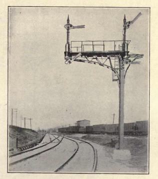
FIG. 13.-Bracket signal.
