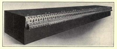
FIG. 93.-Electro-pneumatic interlocking machine.
